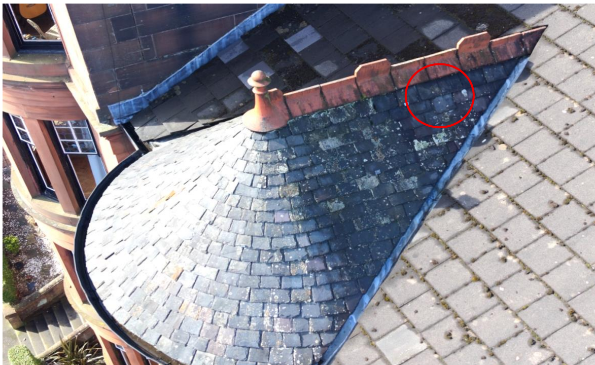
Image 3 (Left bay window, right side) Image shows slipped slate
