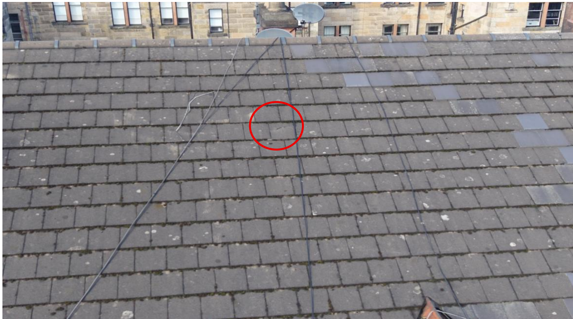
Image 3 (Left bay window, right side) Image shows slipped slate
